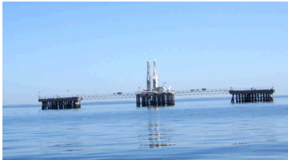
Off Shore Off Loading Platform
